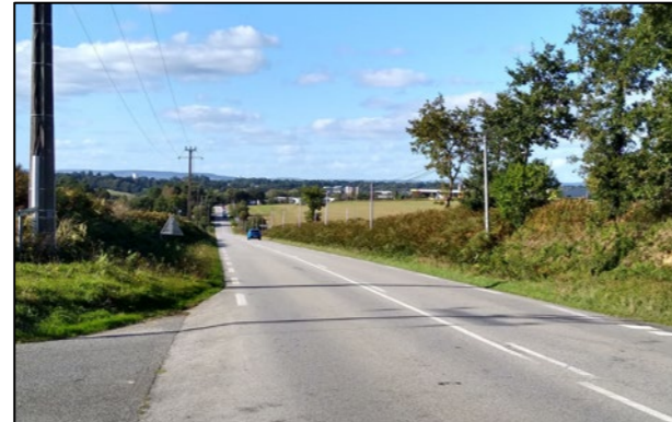
Section Moustoir-Remungol – Pontivy (photo INGEROP)
