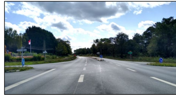
Section Camp de Meucon (photo INGEROP)
