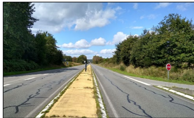
Section Colpo – Locminé (photo INGEROP)
