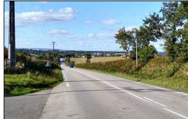
Section Moustoir-Remungol – Pontivy (photo INGEROP)
