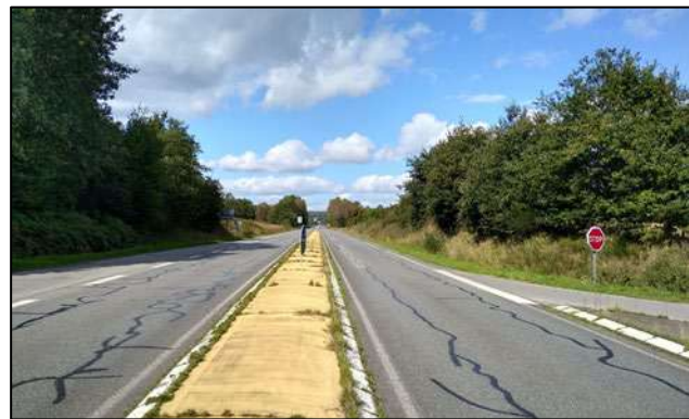
Section Colpo – Locminé (photo INGEROP)
